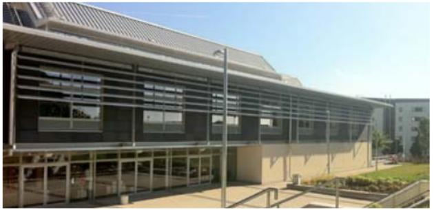
ModCell® frames are made from sustainable FSC and PEFC wood, infilled with locally sourced straw and can be finished with a number of different internal and external finishes. The super-insulated panels, combined with airtight details, mean buildings using ModCell® can meet the demanding PassivHaus specification. This results in zero heat requirements, reduced energy bills and lower CO<sub>2</sub> emissions.
